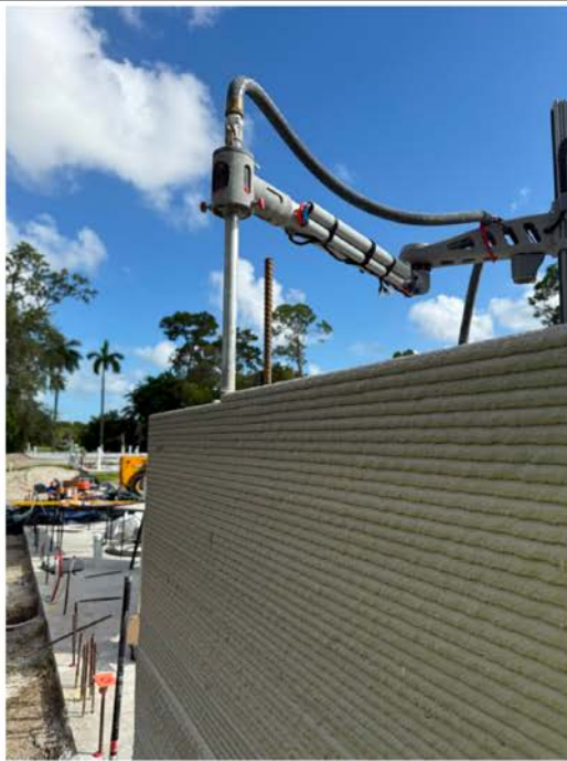
On-site 3D concrete printing — print head laying a continuous wall bead
