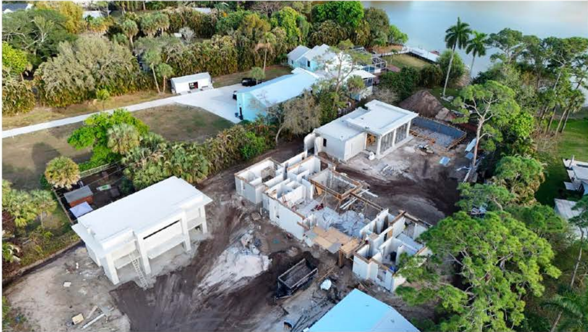
South Florida lakefront residence — 3DCP construction in progress
