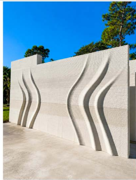
Sculpted 3DCP relief wall — a finish difficult to achieve conventionally
