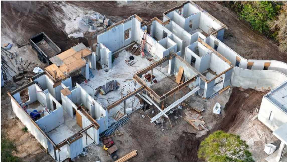
3DCP residence under construction — printed wall system, structure, and site work
