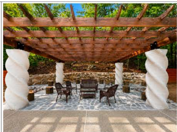
Twisted 3DCP columns — outdoor pergola structure
